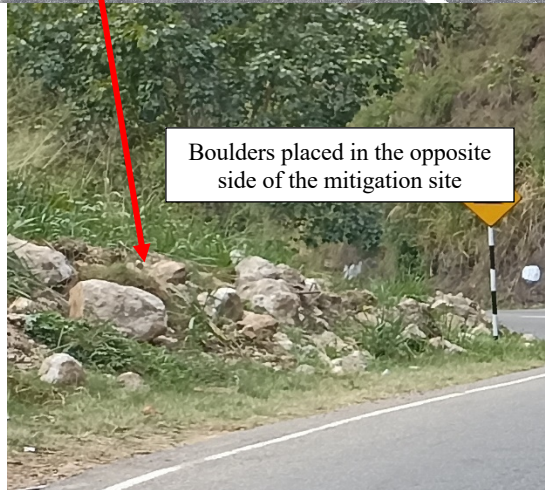
Figure 6a: Ella-Wellawaya (A23) road located adjacent to the cutting failure
